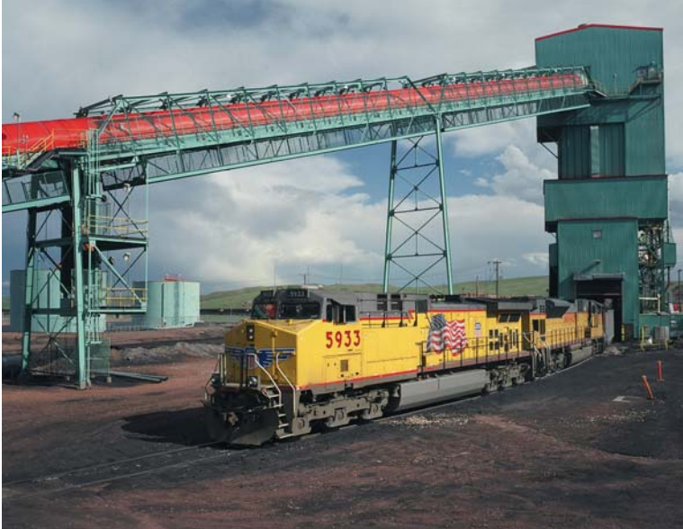
Foundation Energy Belle Ayr mine loads a Union Pacific train.
